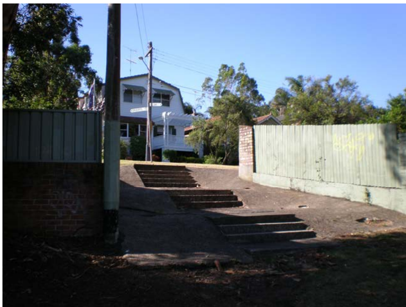
Photo 6: A pedestrian link to Albert Street provides effective off-road access for the students of Hurstville South Public Primary School. Installation of a hand rail is recommended as part of the plan.
