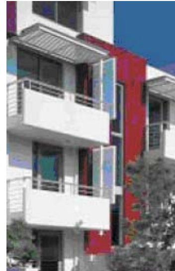
Figure 9. Include sunscreens, pergolas, shutters and operable walls to control sunlight, wind and noise
