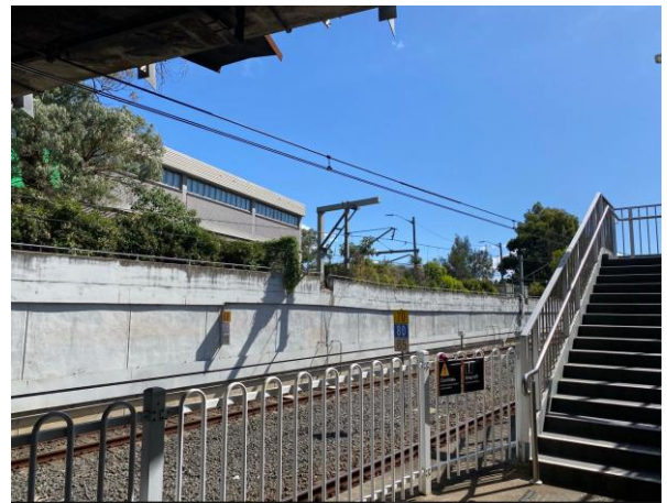
Figure 13 – View of subject site at far western end of station with stairs to access King Georges Road on right.
