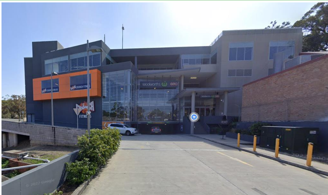
Figure 5: Entry to the subject site from Roberts Avenue
