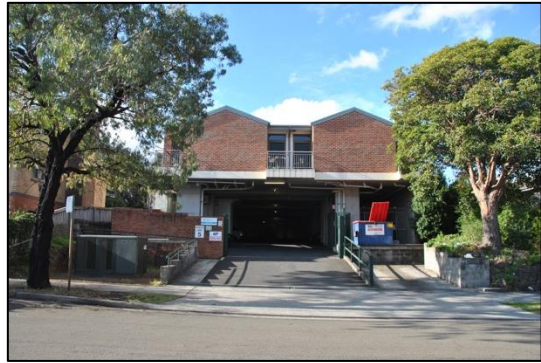
Figure 5 – Site viewed looking North from Millett Street Source: Mecone
