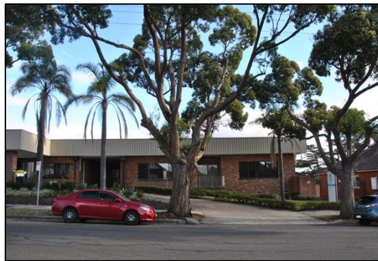
Figure 7 – Site viewed from Gloucester Road Source: Mecone
