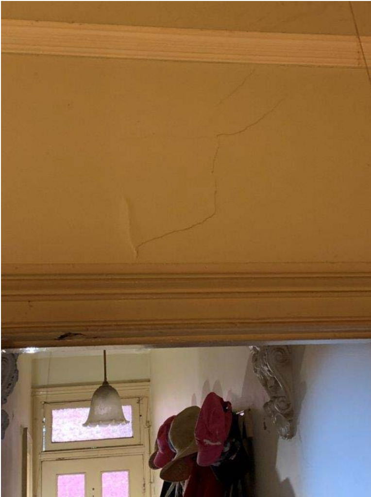
Photo 4 - Cracks in Brick Wall
