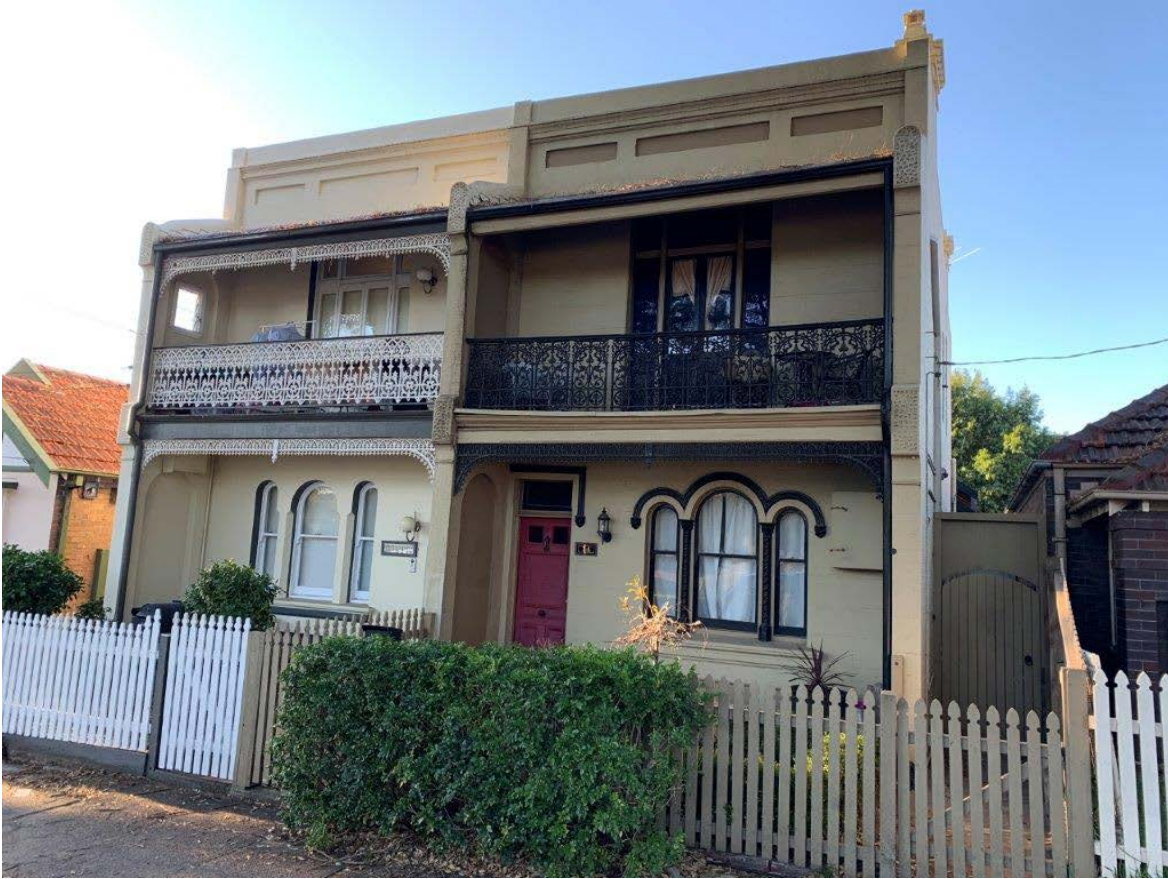
Photo 1 - Overall Photo of 14-16 Victoria Street (Sagging Balcony)
