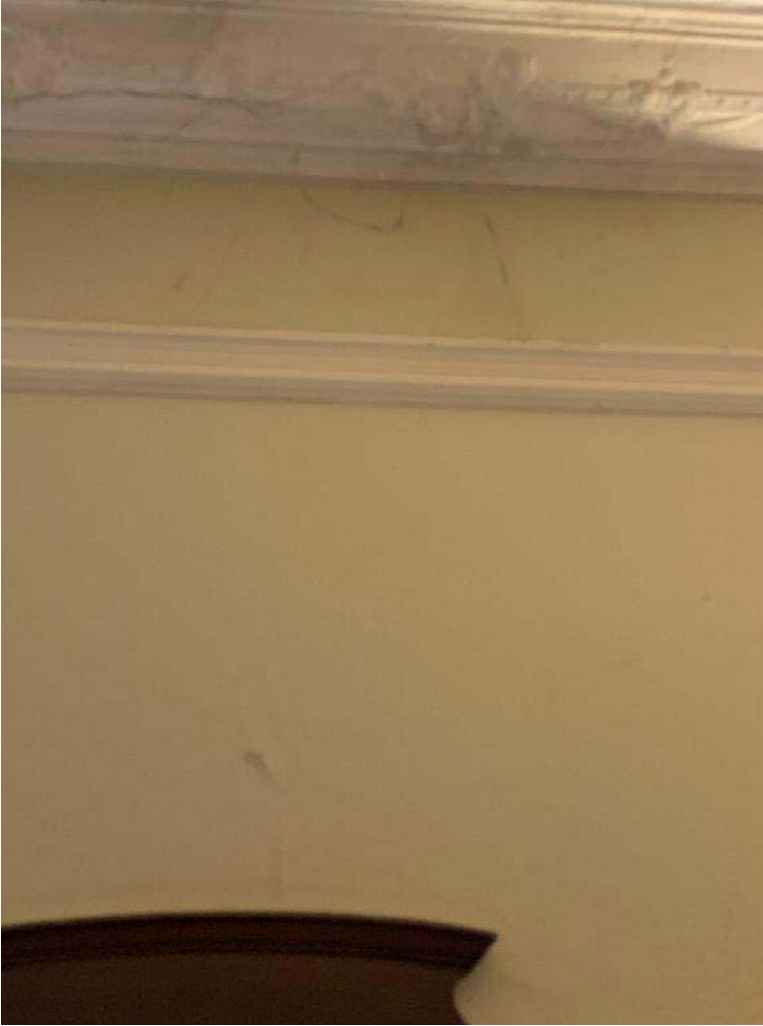
Photo 6 - Cracks in Brick Wall
