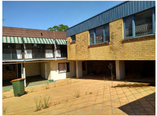
Rear Entry carpark Nursing Home
