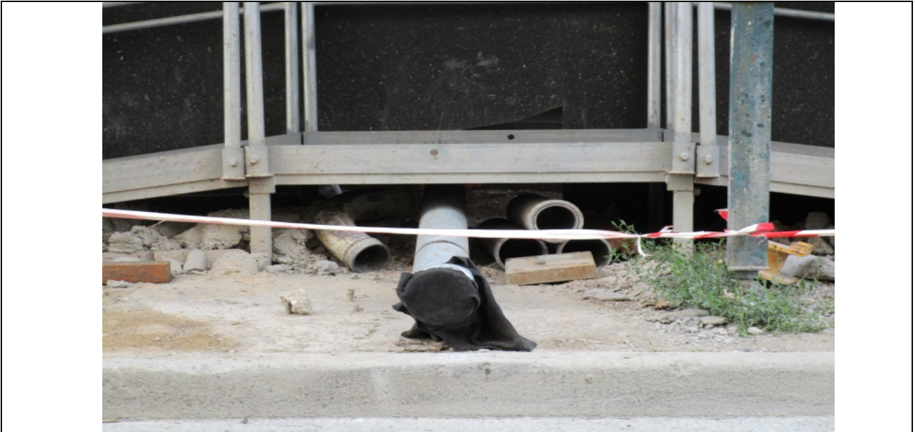
Figures 12 & 13: Pump-line coupling with combined with pedestrian ramp over footway area
