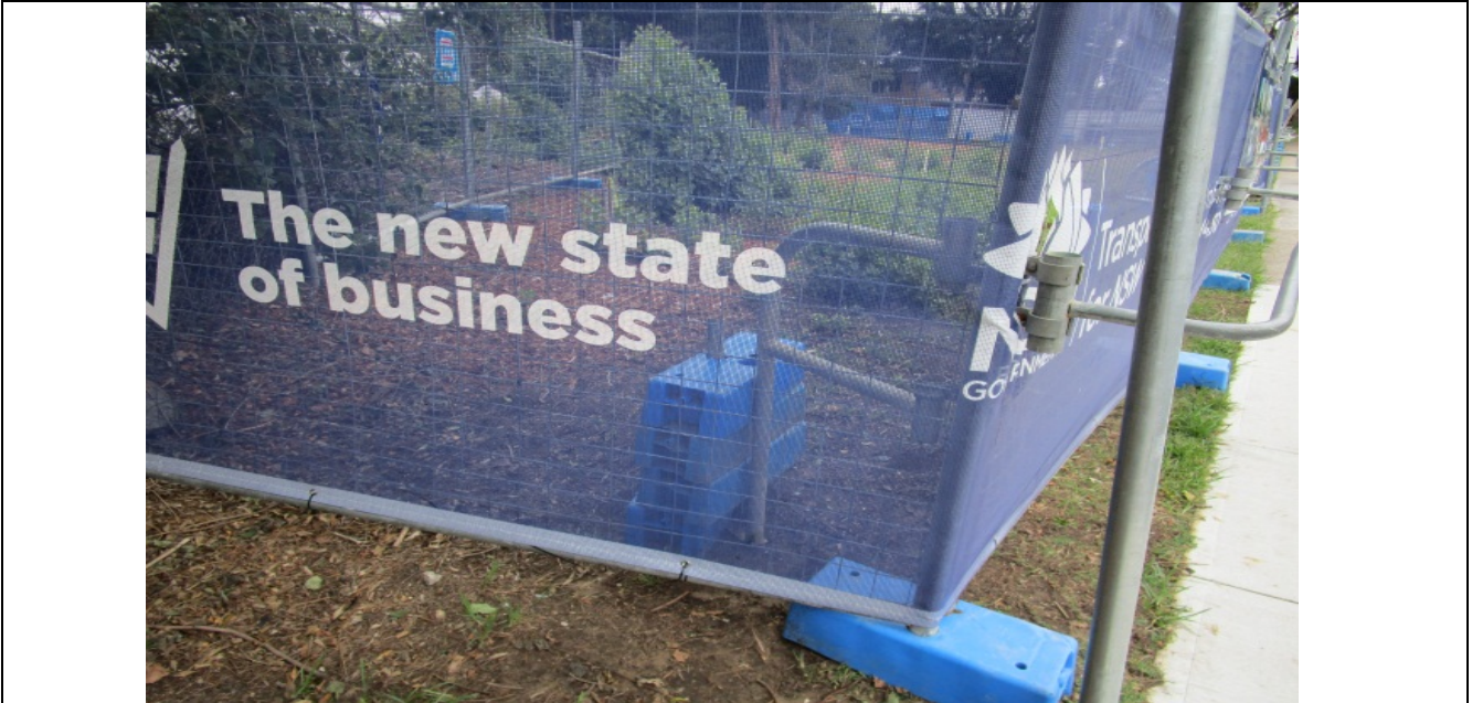
Figure 7: A typical Type C Hoarding – Shade Cloths
