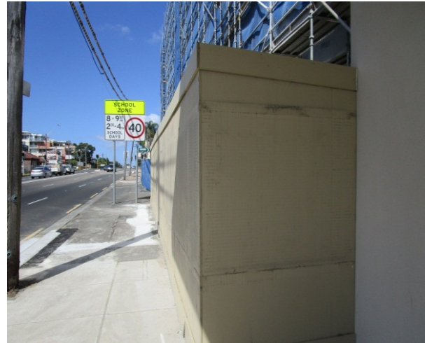
Figures 1 and 2 - Typical Type A Hoarding
