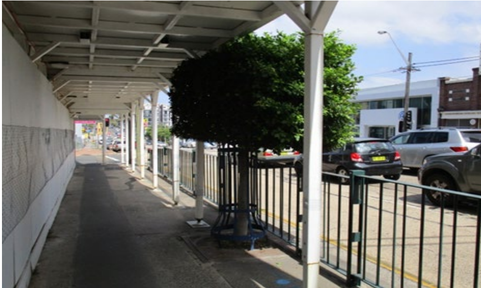
Figure 3: Trunk and limb protection
