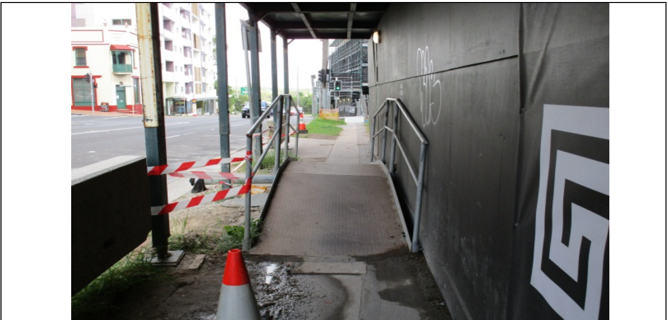
Figures 12 & 13: Pump-line coupling with combined with pedestrian ramp over footway area
