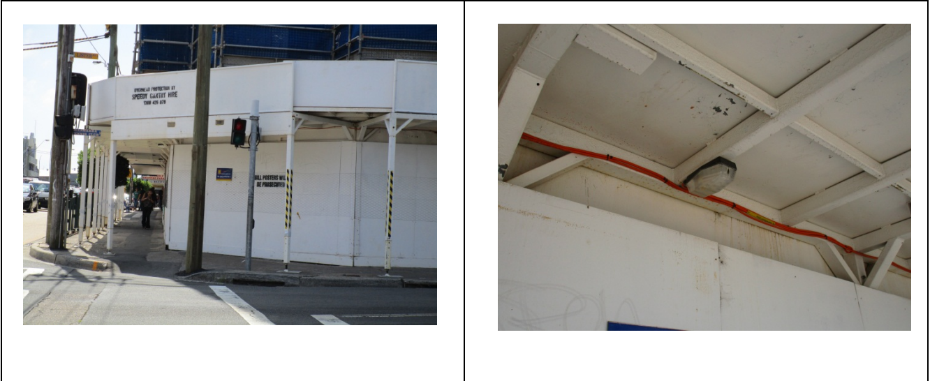
Figures 4 and 5: Typical Type B Hoarding with correction located lighting
