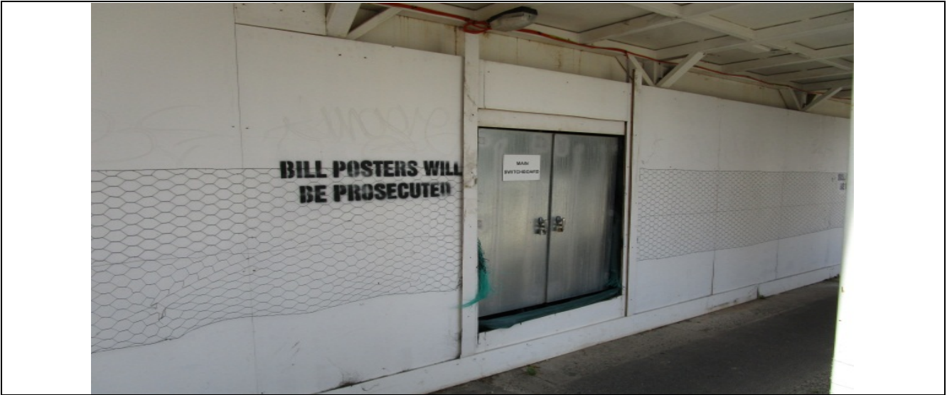
Figure 16: Mesh used to deter bill posters & graffiti
