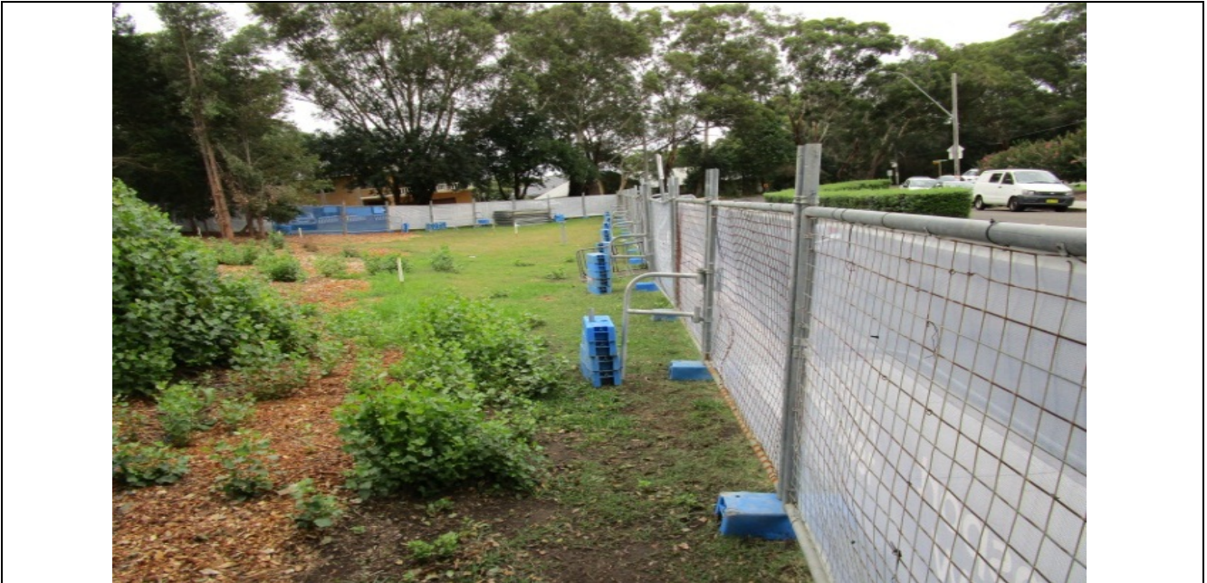
Figure 8: A typical Type C Hoarding – Counter Weights
