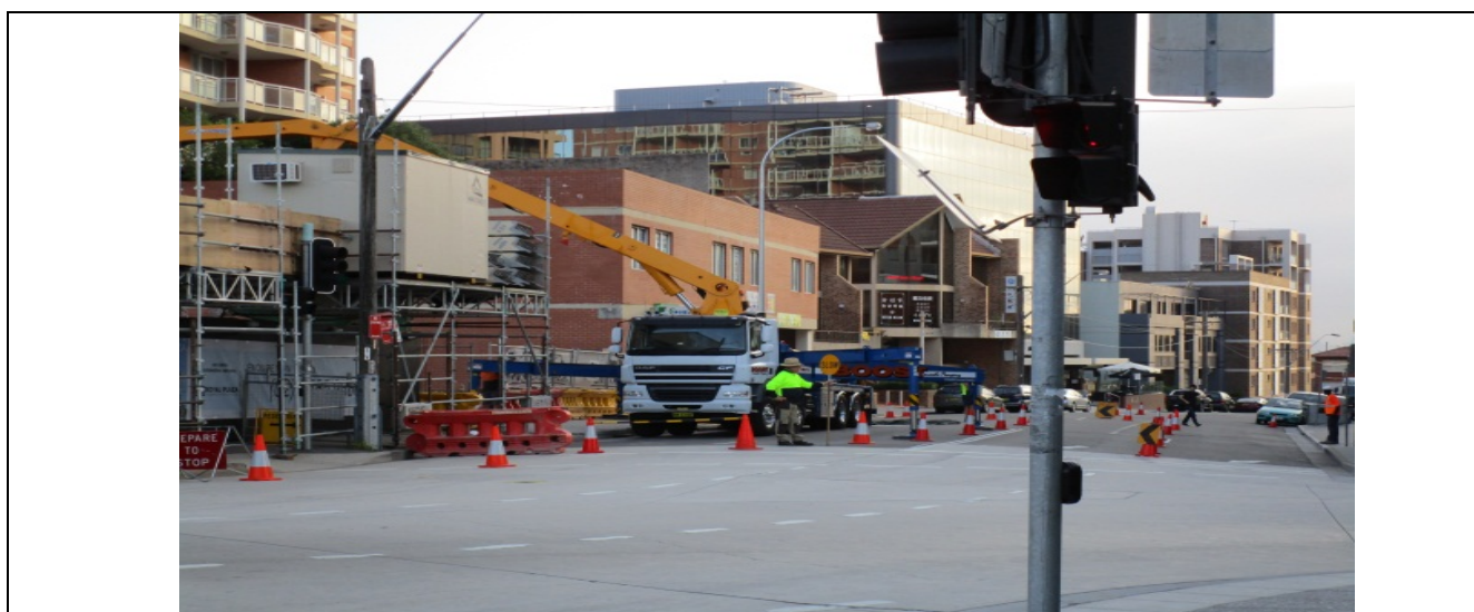
Figure 15: Pedestrian & motor vehicle controllers while hoisting goods.
