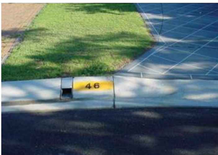
Approved outlet to Council's stormwater drainage system.
