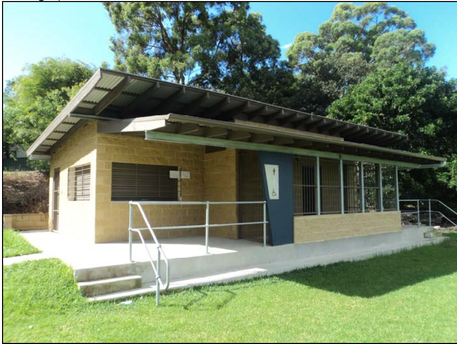
EXAMPLE OF AN ALTERNATIVE SPORTS AMENITIES BUILDING AT QUARRY RESERVE, HURSTVILLE GROVE.
