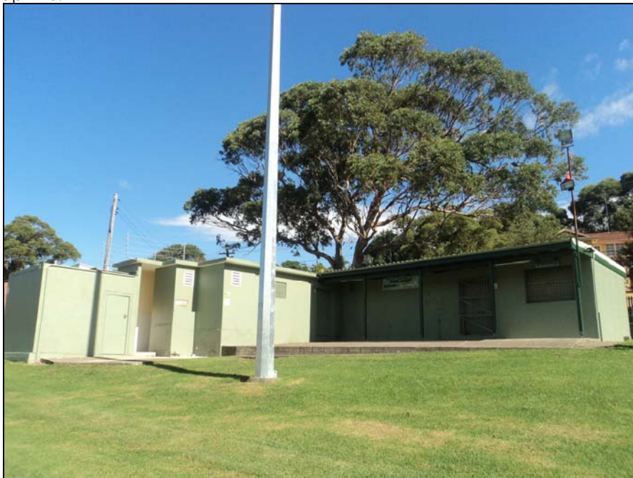
THE GREEN, KYLE BAY PUBLIC AMENITIES BUILDING
