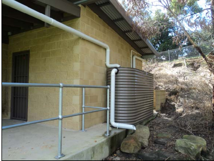
EXAMPLE OF A RAINWATER TANK THAT COULD BE FITTED TO A NEW AMENITIES BUILDING AT THE GREEN
