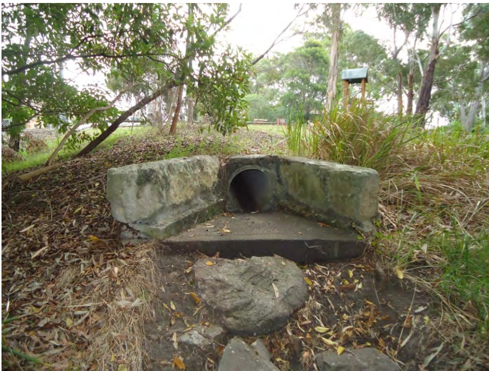
Plate 5 , 'Natural Area - Watercourse' land – Drainage point off Algernon Street
