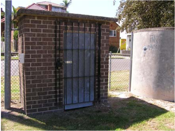
Building and water pumping point
