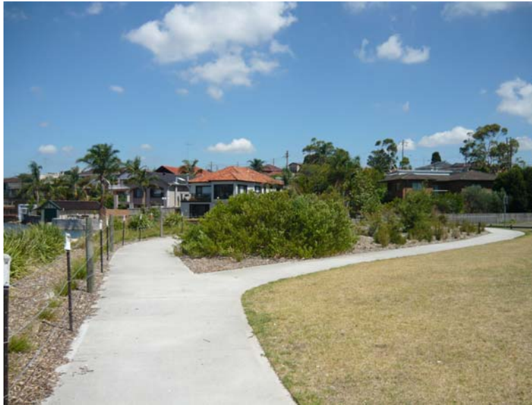
Large bed of native planting to the western end of the sea wall
