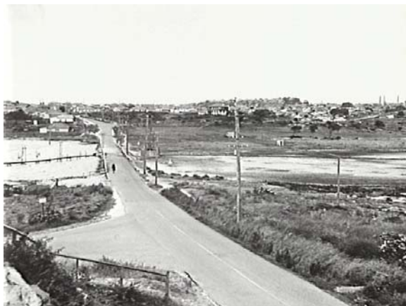
From Ramsgate 1941. The pipeline in Kogarah Bay is carrying silt from the dredging operations in the bay to fill in the swampy areas of the Beverley Park subdivision, including the golf course. The street to the left is The Promenade.
