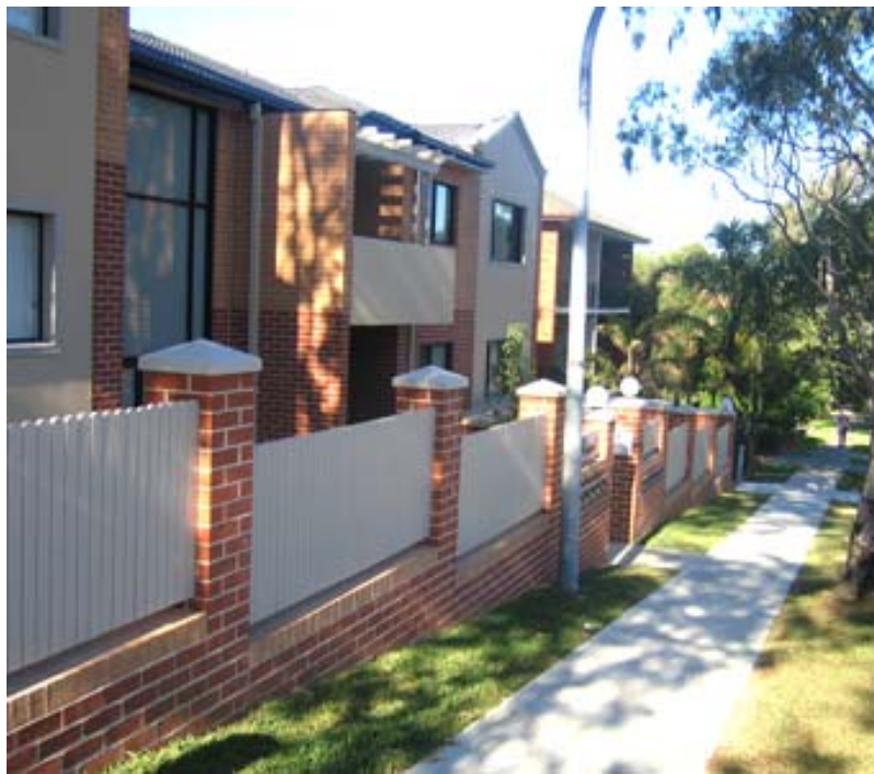
Figure 1. Walls longer than 10 metres must be articulated.
