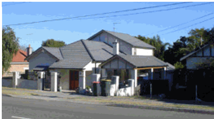
Figure 14. New addition constructed with similar materials and colour palette to the dominant character of buildings in the streetscape.
