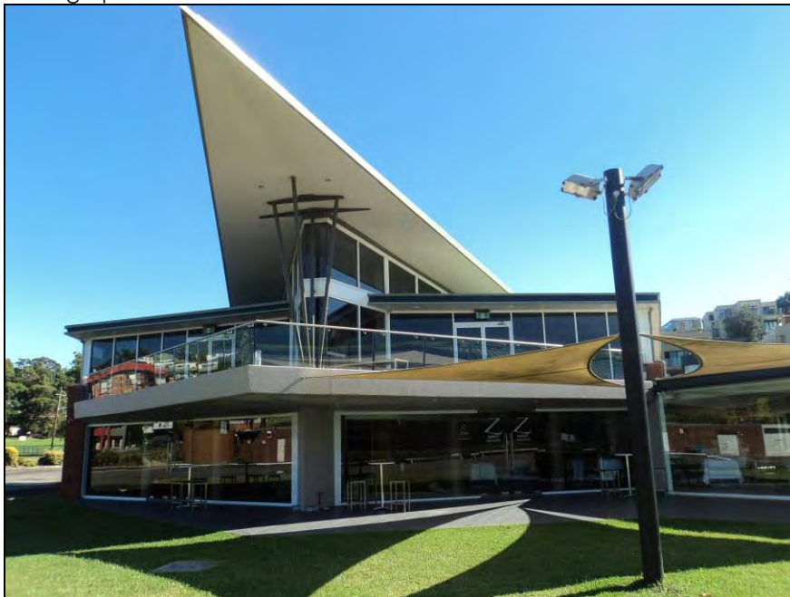
THE KYLE BAY, GEORGES RIVER BUILDING AT MERRIMAN RESERVE.
